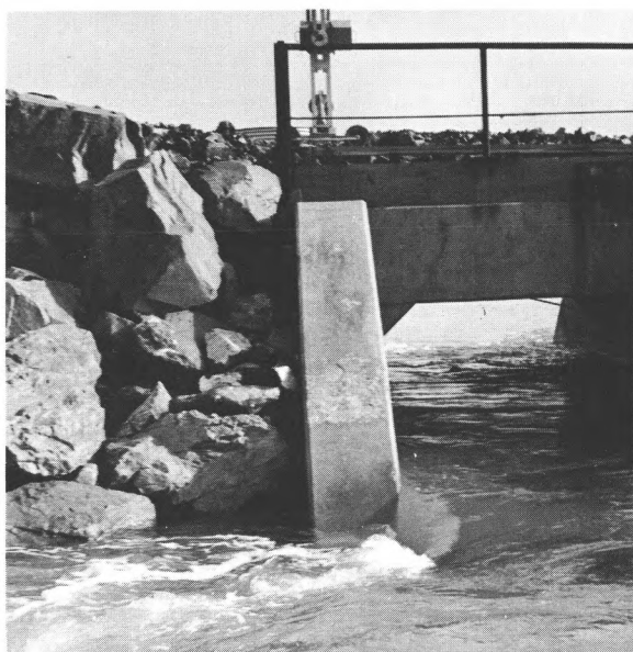
← P 21. Culvert along the Southern Pacific Railroad causeway in the middle of Great Salt Lake. The causeway has divided the lake into two bodies of water, each with its own characteristics. Water rushes through the culvert from south to north inasmuch as the water level in the south arm is more than a foot higher. Evaporation from each body of water is probably the same, but most of the fresh water reaching the lake enters the south arm.
