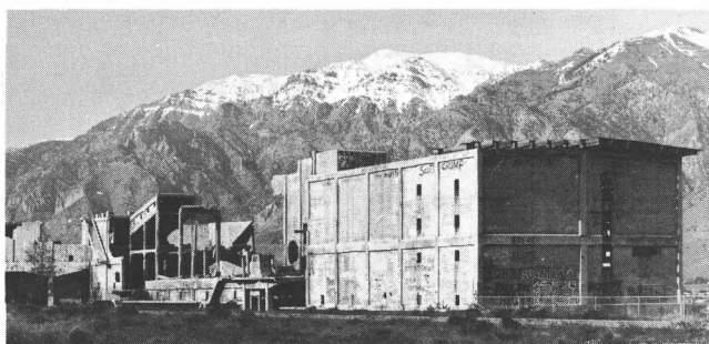
P 31. Ogden Portland Cement Co. plant at Bakers Spur, 5½ miles north of Brigham City (now along Interstate Highway 15). The plant was designed to use marl and clay lying at the bottom of an abandoned lake bed to produce portland cement.
