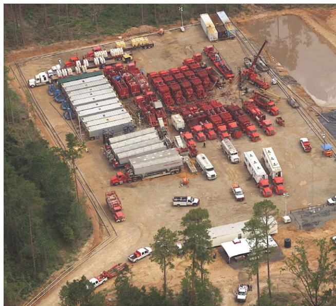
Figure 10.4. Typical frack spread during stimulation treatments in shale. Note pit in the upper right used to store frack water.
