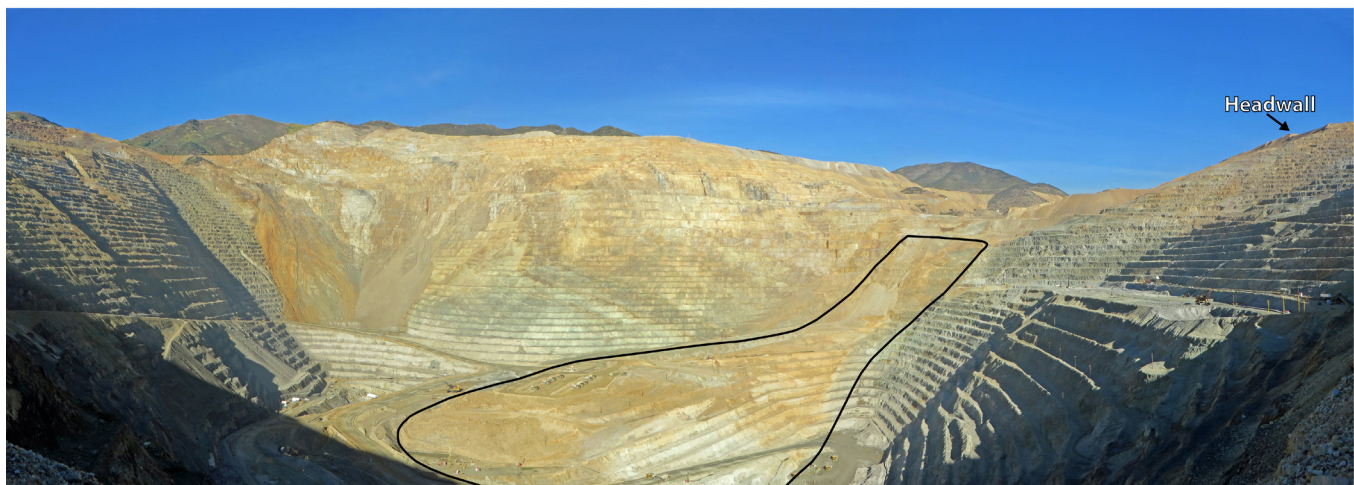
Figure 7. View to the north in the Bingham Canyon open pit porphyry copper-gold-molybdenum mine, taken October 10, 2014. The remnants of the April 10, 2013, 165-million-ton Manefay landslide (rock avalanche) are approximately outlined in the lower portion of the pit. A small part of the 1150-foot high headwall scarp is just visible on the far right-hand margin of the image. For scale, the smallest benches are about 50 feet high.
