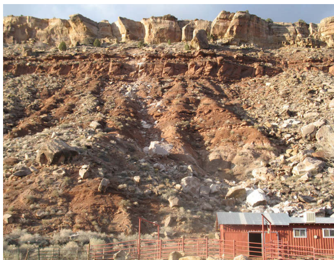
Figure 43. Site showing rockfall source (cliff at top of slope), acceleration zone (steep slope below cliff), and runout zone (base of steep slope near barn and corral). See figure 46 for related information. Photo credit: Dave Black, Rosenberg Associates, photo taken February 2010.
