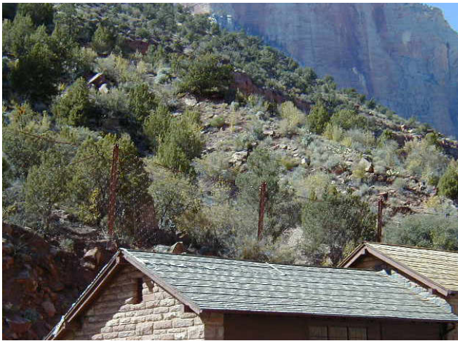
Figure 51. Rockfall fence installed to mitigate the rockfall hazard and protect the Zion National Park maintenance building. Photo taken June 2014.
