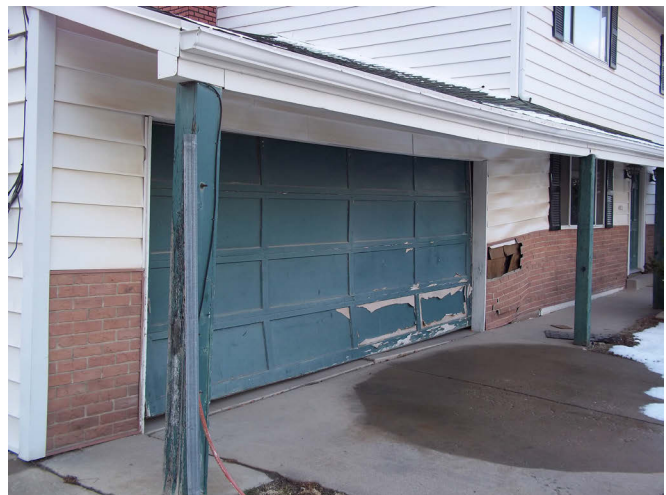
Figure 2. House on Springhill Drive, North Salt Lake City, Utah, severely damaged by the Springhill landslide. This home had been “red tagged” by the city building official as unsafe to enter. Photo credit: Gregg Beukelman, February 29, 2012.
