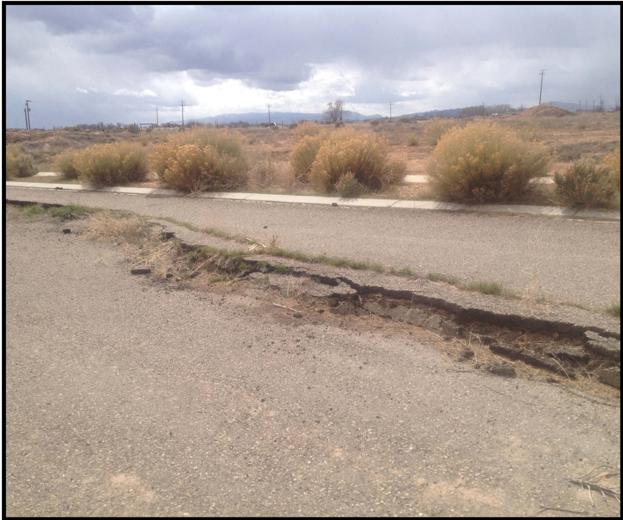
Displacement across an earth fissure that formed in response to groundwater mining in Cedar Valley, Utah.
