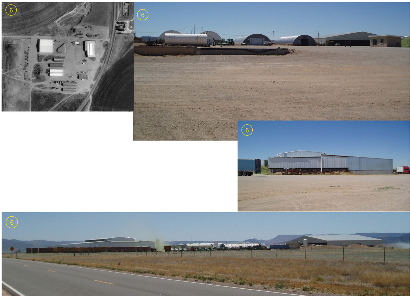
Figure 9. Photographs of a persistent scatterer cluster south of Beryl Junction labeled in figure 5 taken on 6/19/2007.
