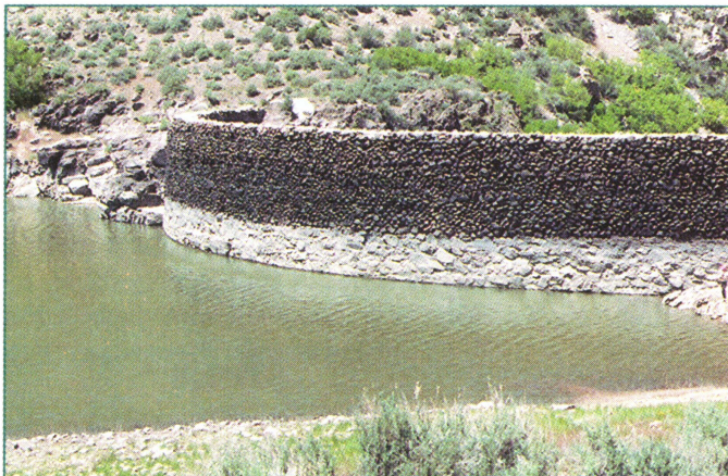
Lower Enterprise Reservoir, shown above, is constructed of rhyolite field stone over slabs of rhyolite dimension stone.
