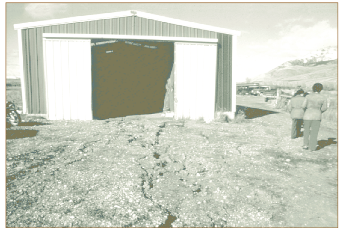
Barn pulled apart one foot at its base by a lateral spread. (Photo courtesy of T. Leslie Youd).
