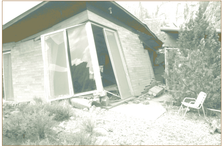
Home damaged in the Springdale landslide that was caused by the 1992 St. George earthquake.
