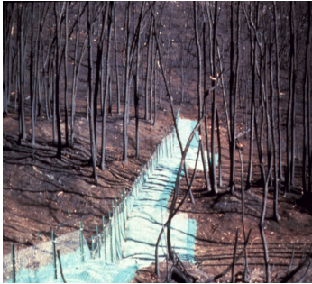
Sediment fence reduces erosion on a wet slope denuded by a wild fire, Freeze Creek, Salt Lake County.
