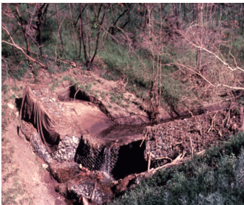
Gabion used to trap debris in Freeze Creek, Salt Lake County.
