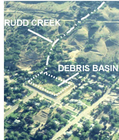
Debris basin in Farmington, Davis County, to trap debris flows issuing from Rudd Creek.
