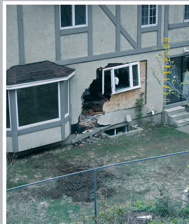
Boulder that bounced downslope through the back of a house (above-left) came to rest in the garage (above-right) after falling through the floor. Provo, Utah County, Utah, April 2009. Photo Credit: Provo Fire Department.
