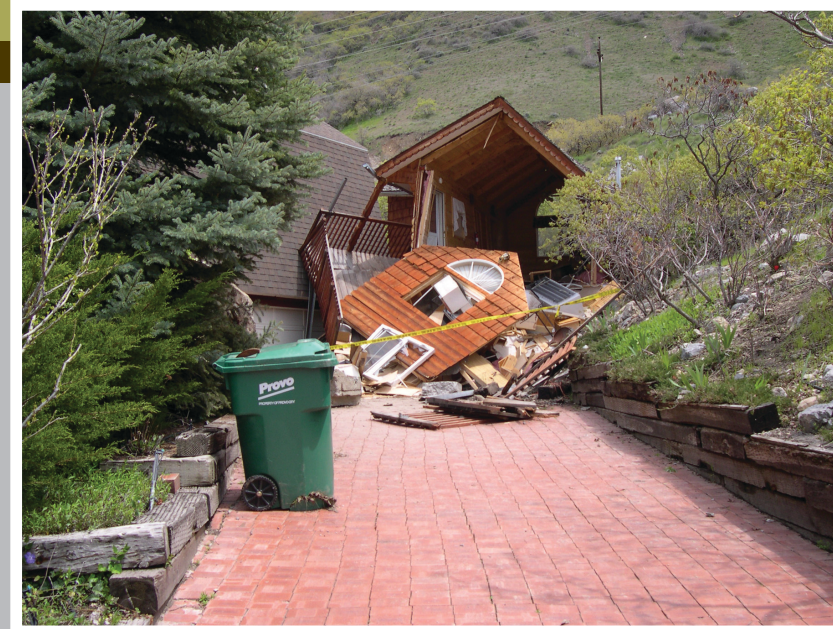
A large boulder destroyed a guest house (above-left) before the boulder stopped next to a large tree (above-right), Provo, Utah County, Utah, May 2005.
