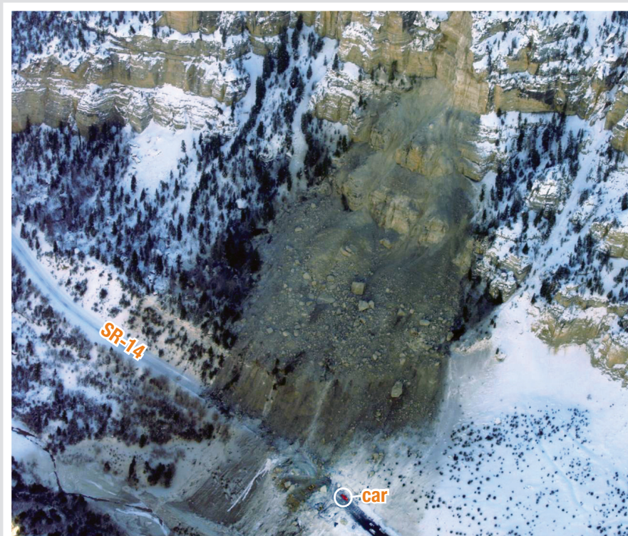
Rock slide closed SR-14 in Cedar Canyon, Iron County, Utah, January 2009. Photo credit: Mel Aldrich.
