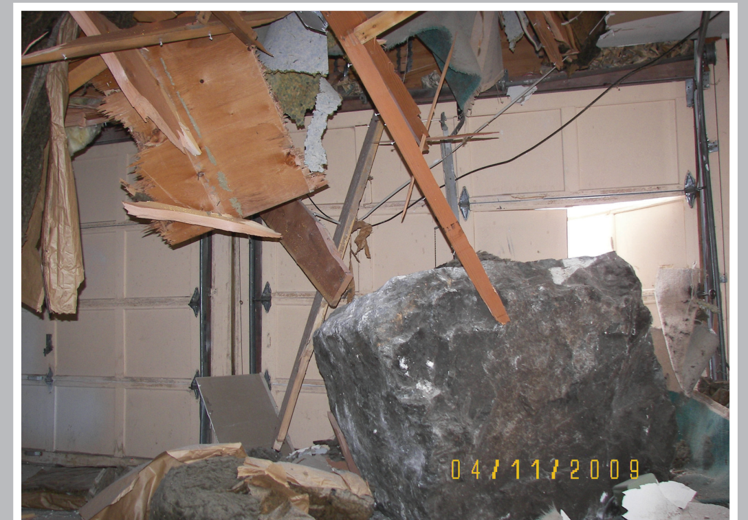
Boulder that bounced downslope through the back of a house (above-left) came to rest in the garage (above-right) after falling through the floor. Provo, Utah County, Utah, April 2009. Photo Credit: Provo Fire Department.
