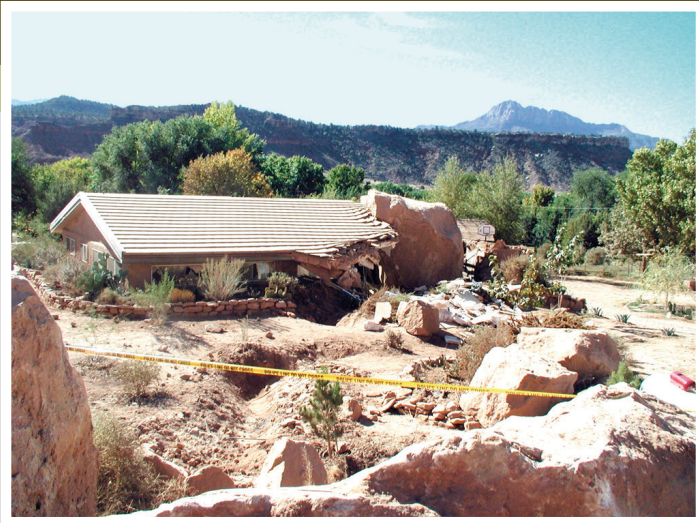
Boulder detached from the north wall of Zion Canyon, estimated to weigh 300 tons, damaged this house in Rockville, Washington County, Utah, October 2001.
