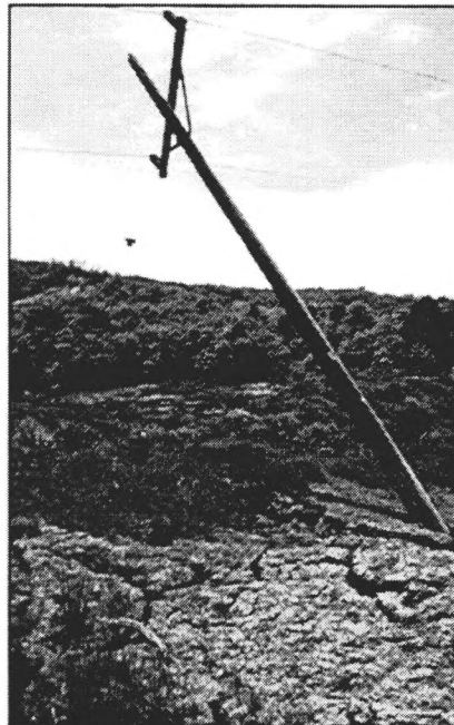
Figure 3. Transmission pole tilted by landslide movement. Pole is one of two in upslope set of Utah Power & Light (UP&L) transmission poles on landslide. Downslope movement caused one of three powerlines to be severed from pole. Powerlines were subsequently abandoned by UP&L.
