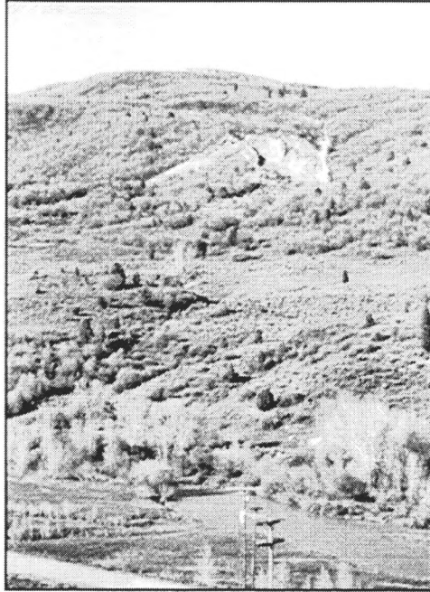
Figure 2. The Shurtz Lake landslide on May 9, 1997. View is to the south from Utah Highway 6. Spanish Fork River is visible in bottom of photograph.
