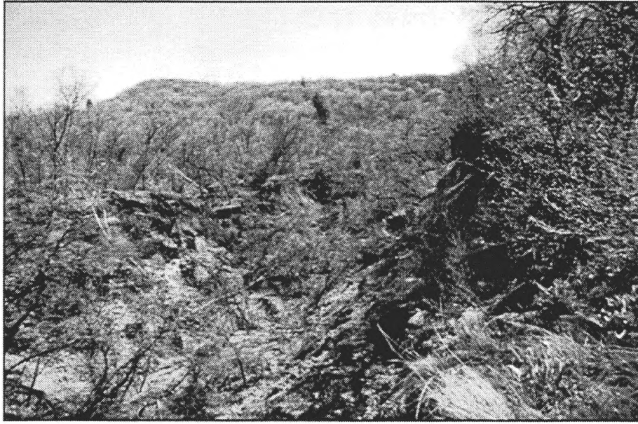
Figure 16. Slumping along the left-flank gully upslope of the crown of the left-flank earth flow. View is to the south.
