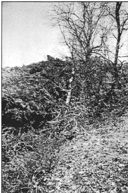
Figure 4. Lateral levee along northwestern edge of left-flank earth flow. Levee is about 10 to 15 feet high.
