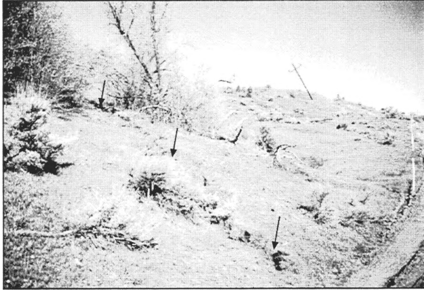
Figure 14. Right-lateral scarp (arrows) upslope of power-line access road. The ground surface on north side of scarp is heaved upward several inches. Note tilt of transmission pole. View is to the west-northwest.
