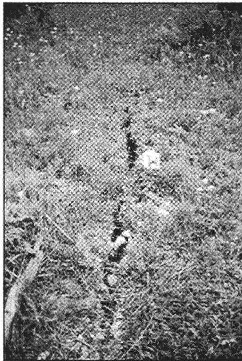
Figure 21. Ground crack observed on May 30 over 200 feet downslope of May 7 toe of landslide. Deformation suggests distribution of landslide activity is enlarging and progressing downslope. Cracks likely formed following heavy precipitation over the Memorial Day weekend. Field book is about 7-1/2 inches long.
