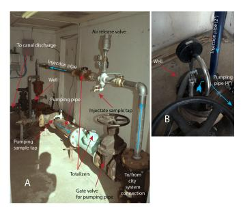
Figure 13. Configuration of the Glenridge well house for Millville's ASR program. A) View of inside of Glenridge well house. Connection to Millville's culinary system is in foreground and the well is in the background. B) Close-up view of well head.
