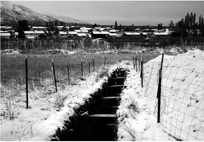
Figure 8. South (downslope) view of the Harrisville trench excavated on the flank of a hummock.
