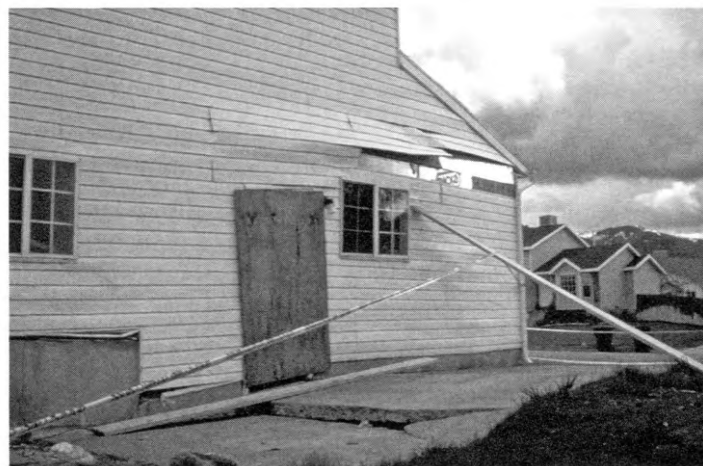
Severe damage to a house on the Sunset Drive landslide, Layton, April 1998. House was subsequently condemned by Layton City and demolished.
