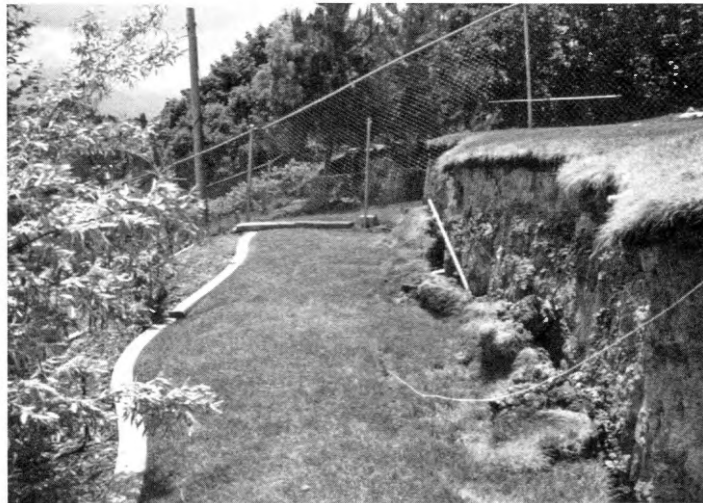
Landslide damage at a lot on Capitol Boulevard, Salt Lake City, June 1998. Landslide movement formed a scarp and offset the backyard of the home by more than 5 feet. Fence in background and underground piping to sprinkler system were damaged by movement.
