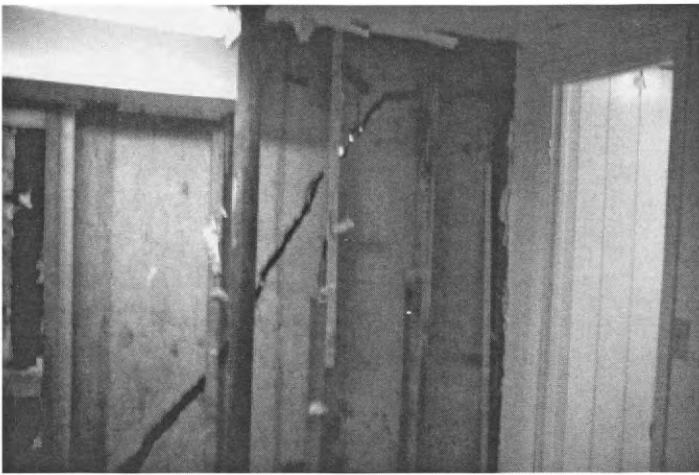
Large crack developed in a concrete foundation wall on Springhill Circle. Wall board has been removed to expose crack. Outside light can be seen through the upper portion of the crack.
