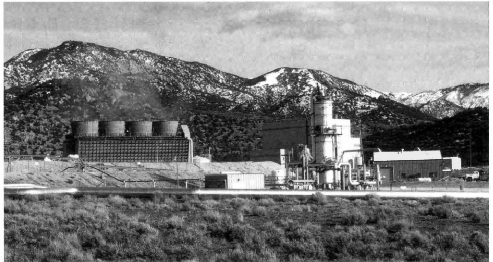
Utah Power's Blundell geothermal power plant at Roosevelt Hot Springs geothermal area near Milford: cooling stacks and power plant building, with the Mineral Mountains in the background. View is to the southeast.
