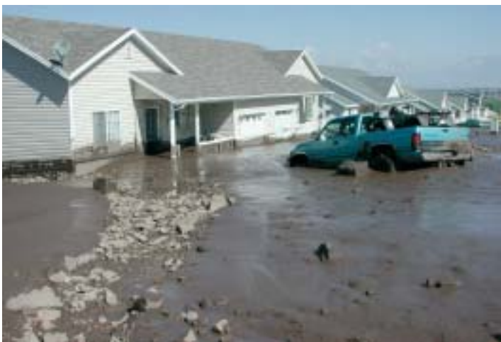
The debris flow entered the front and garage doors of this house on Peach Street in Santaquin.
