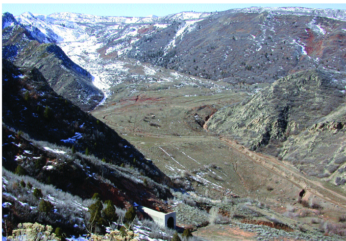
Thistle landslide, February 2005. View to the west from pullout on U.S. Route 6/89. Note railroad tunnel at bottom center (constructed after the landslide buried the original railroad grade).
