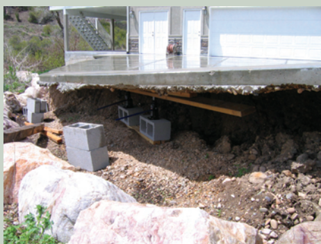
Landslide movement left this concrete driveway slab suspended in the air in the Creekside Drive area, Mountain Green.
