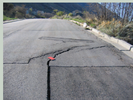
Damage to road in upper part of Sherwood Hills landslide, Provo.
