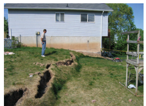
This house at 1843 East Sunset Drive straddles the main scarp of the landslide. Landslide movement has removed support from beneath part of the foundation.
