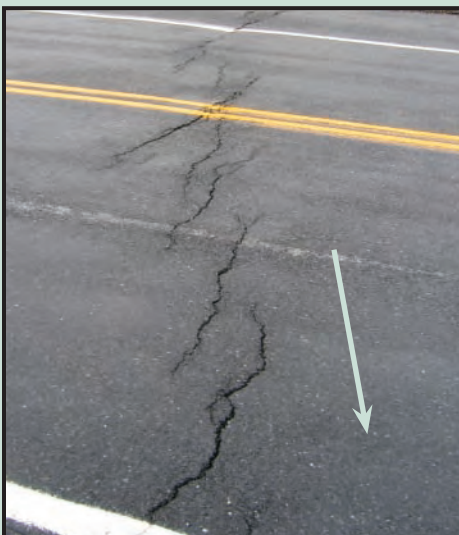
Road cracks across State Route 226 define the edge of the Green Pond landslide. Arrow is on slide and shows general movement direction.
