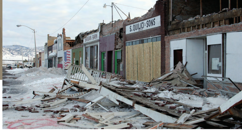
Unreinforced masonry buildings in the historic district of Wells were severely damaged in the earthquake.
