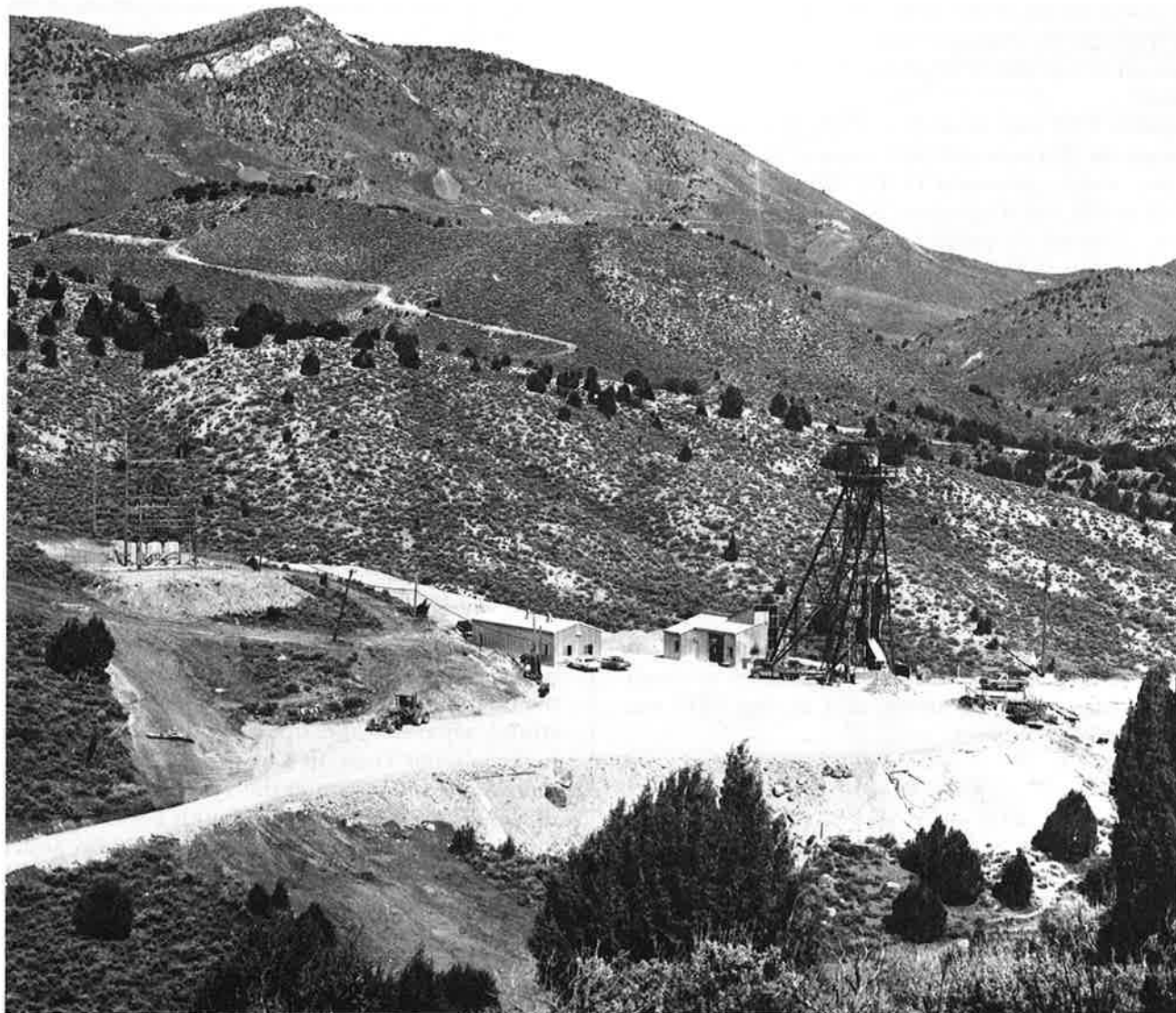
FIGURE 67. — Surface installations of Trixie mine. Dumps in left background mark mines of Iron Blossom ore zone of main Tintic district.
