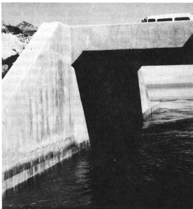
B. View of one of the culverts in the causeway. Depth of water in culvert is about 10 feet. Upper few feet of water is moving northward away from viewer; lower lower few feet is moving southward. (Photograph by D.C.Hahl, 1964.)
