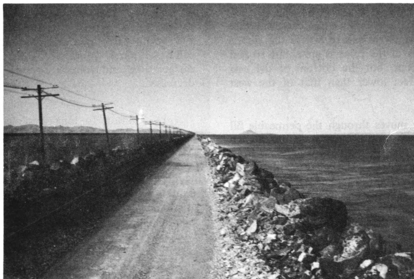
A. Overall view of the causeway across Great Salt Lake. Dark line on left side of photograph at the base of the mountains on the western margin of the lake is the trestle of the former railroad crossing. (Photograph by D.C.Hahl, 1964.)
