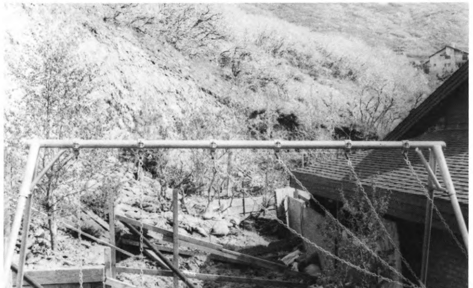
Slope failure of colluvium behind home along mountain front in Salt Lake City. Note projective measures with debris against house.
