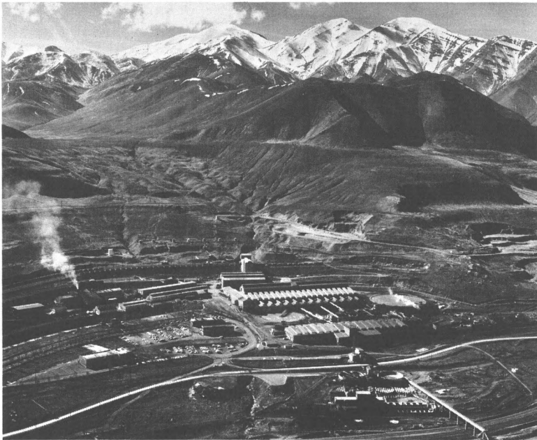
Figure 53. View looking westerly across the Arthur concentrator of the Kennecott Copper Corporation, Salt Lake County, Utah. Note the prominent Lake Bonneville beach terraces in the middle background.
