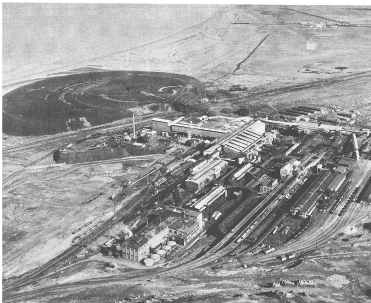
Figure 54. View looking northeasterly across the Garfield smelter, now known as the Utah Smelter of the Kennecott Copper Corporation, Salt Lake County, Utah. Note slag dump in left background and also the plant of Western Phosphates in upper right corner.
