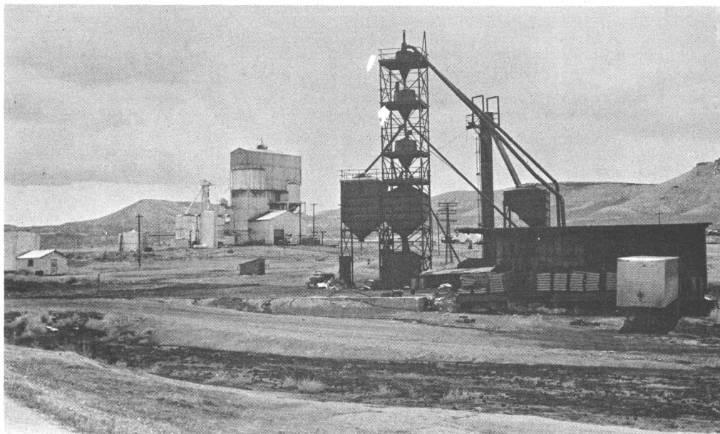
Figure 7. View of the mining and treatment facilities of the American Gilsonite Company at Bonanza, Utah. This highly mechanized mine area is in contrast to the other small mines in the gilsonite area. The shed in the foreground contains 100 pound paper bags of gilsonite ore ready for shipment.
