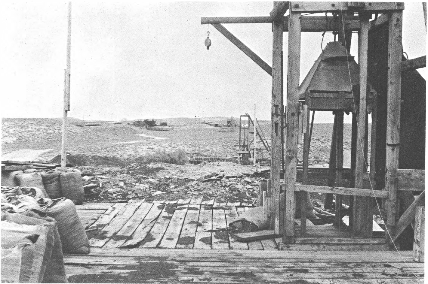
Figure 10. Small mines on the Bonanza vein, near Little Bonanza. The three shafts in a straight line indicate the strike of the vein. Gilsonite ore in 200 pound burlap bags stands nearby ready for shipment to buyers. This picture is a good illustration of the mining practices employed in these small mines. The ore is crushed and reduced to a fine powder.
