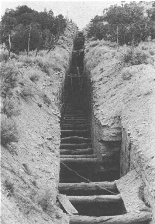
Figure 9. The Pride-of-the-West vein, west of Rainbow, Utah, showing how the firm vein walls are supported by wooden stulls with practically no caving. Note the small offset in the right vein wall and the fact that the walls are clean of gilsonite. This view is looking along an old mining and hauling level, as evidenced by the supporting stulls all on the same level. The plank flooring has been removed. (Photograph by Don Preston)
