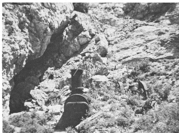
P-3 Open stope in metamorphosed dolomitic limestones, mined in the Highland Chief-Wellington workings, Prince of Wales Hill, in the 1870s. Machinery is steam powered compressor, probably the first in Utah.
