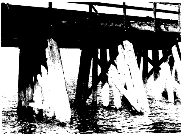
Figure 2. Pilings used on original causeway. Photo by David Miller.
