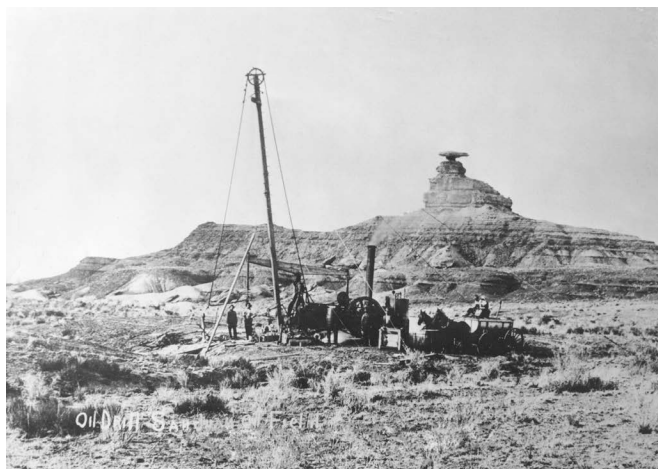
Figure 1.6. Cable-tool drilling near Mexican Hat, San Juan County, Utah, circa 1920. Used by permission, Utah State Historical Society, all rights reserved.
