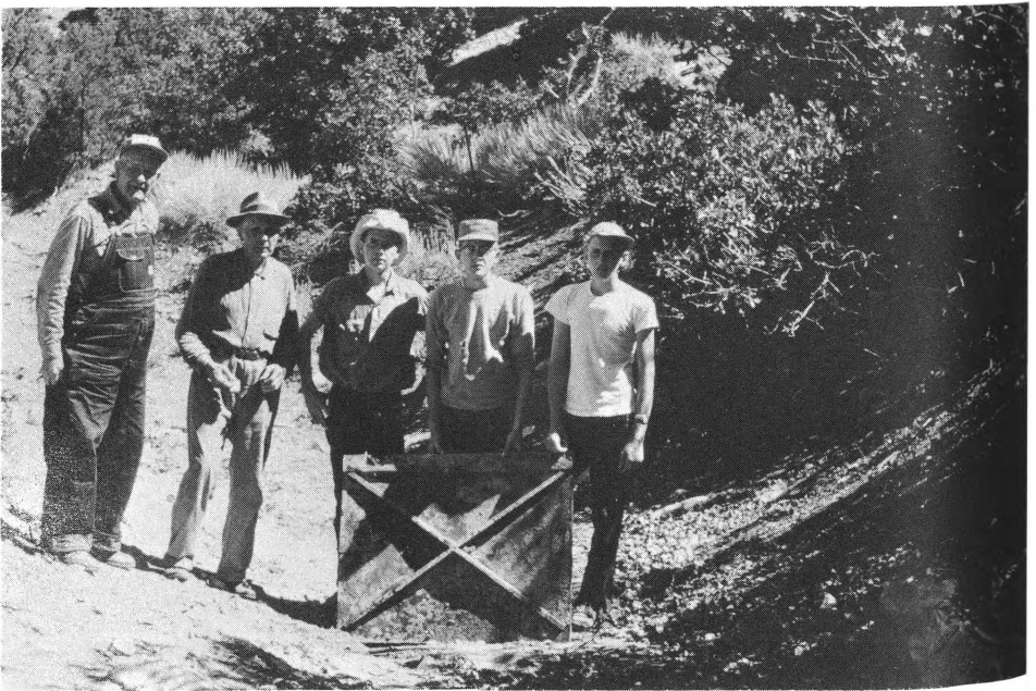
Figure 5. J. E. Hanson, Alms C. Dalby, Carl Dalby, Richard Dalby, and Alen Dalby standing behind a \frac{3}{4} inch thick x 2\frac{1}{2} feet x 3\frac{1}{2} feet cast iron plate. This probably represented the floor of the retort. Though separated from the round lid shown in figure 4, this rectangular plate was down stream from the old retort site which had not been discovered when this picture was taken.
