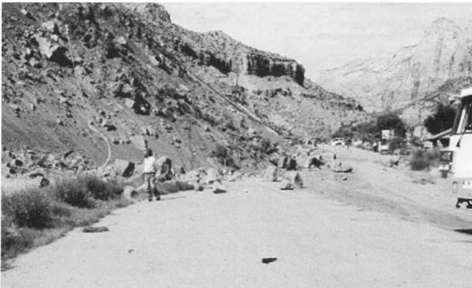
Figure 5. Toe of the Springdale landslide near State Route 9. Note ruptured utility lines in the toe of the slide. Photo by B.D. Black.
