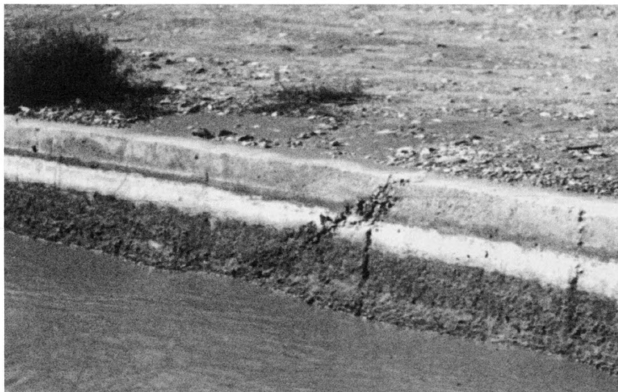
Figure 7. Cracks in the concrete lining of the Shinob Kibe canal.
