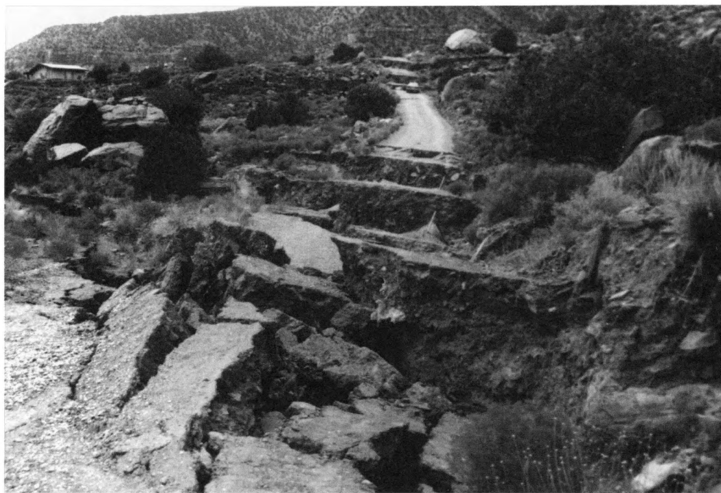
Figure 6. Graben extending parallel to direction of landslide movement (right to left). The car (visible in the upper center) was abandoned by homeowners trying to escape the landslide; the road was blocked by the far wall of the graben, which must have formed before the near wall (foreground).
