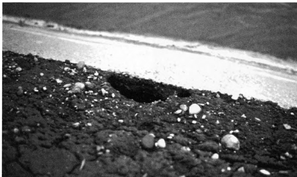
Figure 8. Cracked lining and piping along the Shinob Kibe canal.
