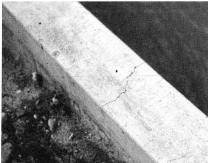
Figure 5. Crack in a wing wall of the Washington Fields diversion dam.
