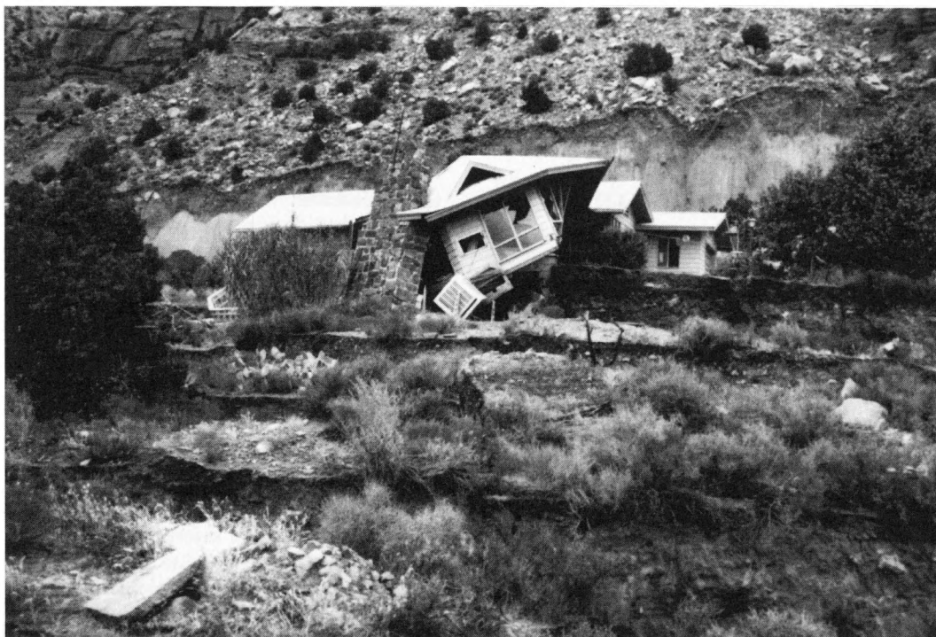
Figure 7. House on the western part of the Springdale landslide destroyed by differential movement along internal scarps and other fractures. Main scarp is visible behind the house.
