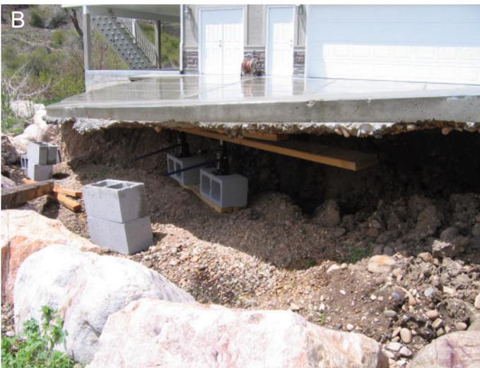
**Figure 6.** A) Damage caused by movement of the main Creekside Drive landslide in Mountain Green forced abandonment of this house. B) On Cascade Drive, Mountain Green, landslide movement left this concrete driveway slab suspended in the air.
