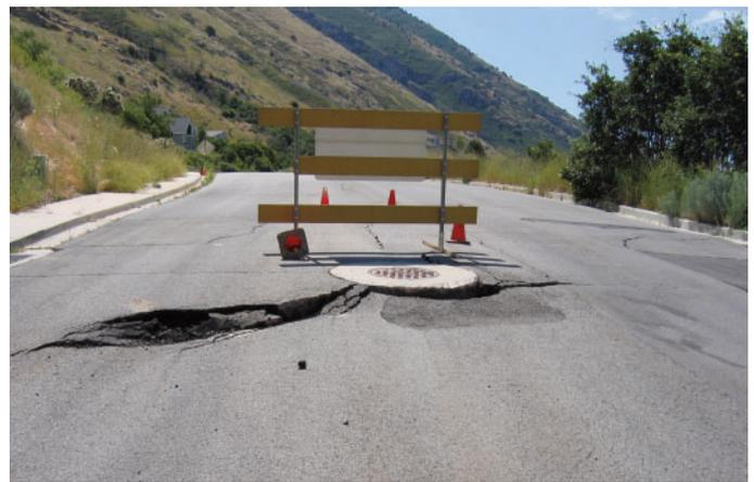
**Figure 7.** Damage to road in upper part of Sherwood Hills landslide, Provo.
