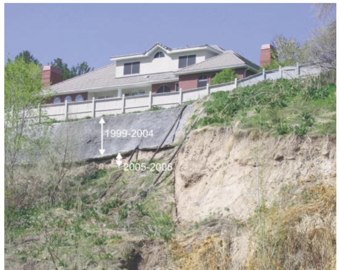
**Figure 8.** Offset on main scarp by repeated landslide movement, City Creek Canyon, Salt Lake City. Concrete covers the main scarp that formed between 1999 and 2004. Fresh soil is exposed below due to continued movement in 2005 and 2006.
