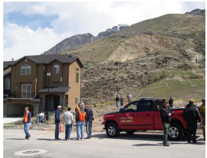
Figure 2. Damaged townhouse building and disrupted toe and main scarp of the landslide in Cedar Hills.
