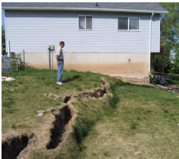
**Figure 5.** This house at 1843 East Sunset Drive in Layton straddles the main scarp of the landslide. Landslide movement removed support from beneath part of the foundation.
