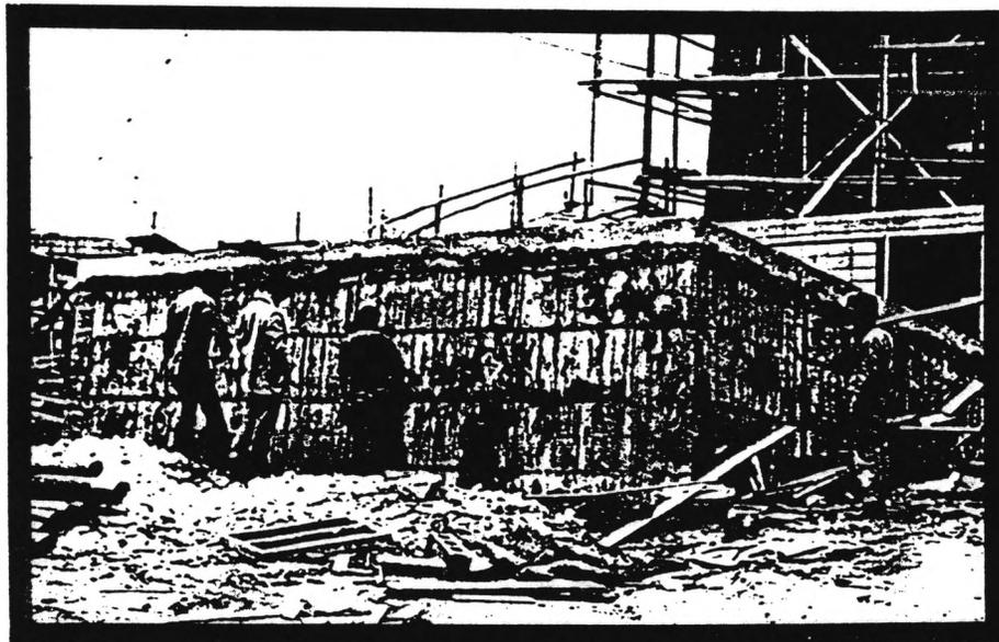
**Figure 15.** Sewage treatment tank floated to ground surface during 1964 Niigata earthquake (after Seed and Idriss, 1967).
