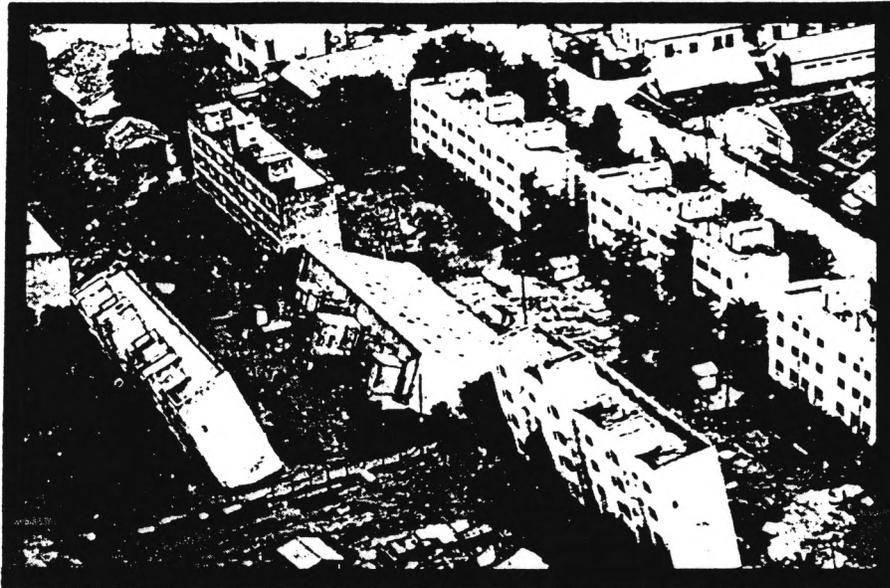
**Figure 14.** Tilting of apartment buildings during the 1964 Niigata earthquake (after Seed and Idriss, 1967).
