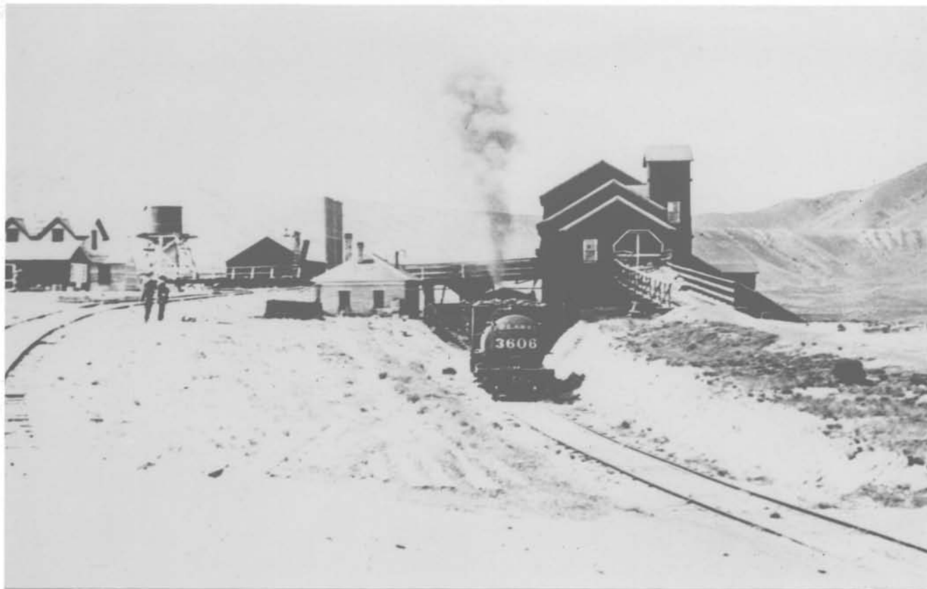
8. An early view of the Bauer mill, looking south toward Stockton Bar, and trackage of Union Pacific Railroad Mill was first known as the Bullion Coalition gravity concentrator, built for the Honerine mine in the Stockton district. This was accessed by a long drainage tunnel east of the mill. It was purchased in the 1920s by Combined Metals Reduction Co., partially to treat ores brought by railroad from Pioche, Nevada. Later it was converted to flotation.
