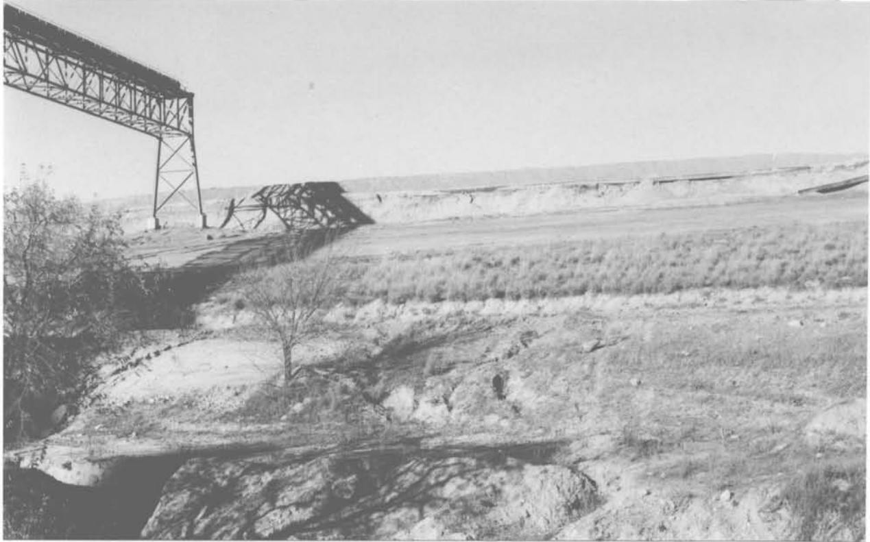
14. Some of the extensive Kennecott copper tailings, shadowed by the frame of an old conveyor gallery, near Magna, Salt Lake County, 1987, prior to reopening of operation. Parts of the Magna and Arthur plants have since been closed permanently.
