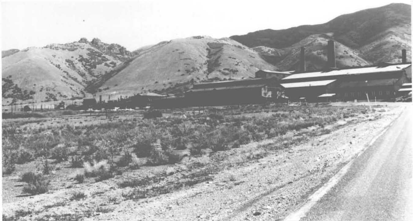
4. Part of Tooele smelting plant (mainly the copper smelter; plant office to left). Some of the heavy equipment was brought from Anaconda's former Washoe Copper Co. plant at Anaconda, Montana, probably via an earlier smelting installation west of Murray.
