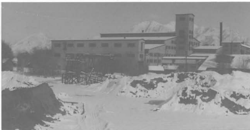
11 and 12. Closer views of main flotation building, United States mill, Midvale. Plant is briefly described by Nackowski, 1964. The heavy concrete construction of this and other plants of the era suggests the faith company personnel and investors had in the future of Utah's base metals industry.
