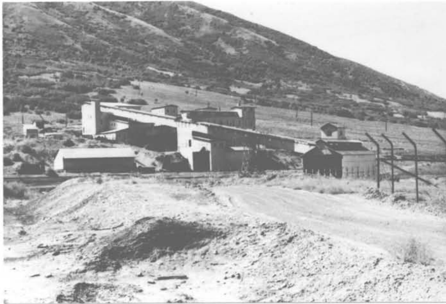
Fig. 3. One of two mills at the former Tooele smelting plant, International, Tooele County. Ore from distant mines arrived by railroad, while ore from Bingham arrived by an aerial tramway extending over the Oquirrh range. Plant was dismantled in 1976; one conveyor gallery was incorporated in building Trolley Square, Salt Lake City.
