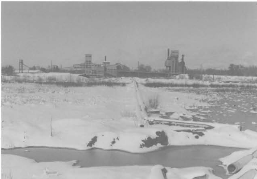
10. United States (U V Industries or Sharon Steel) mill and tailings near Midvale, Salt Lake County, 1982. Railroad (center) brought non-porphyry ores from Bingham district for processing by selective flotation. The mill also treated custom ores from other districts.
