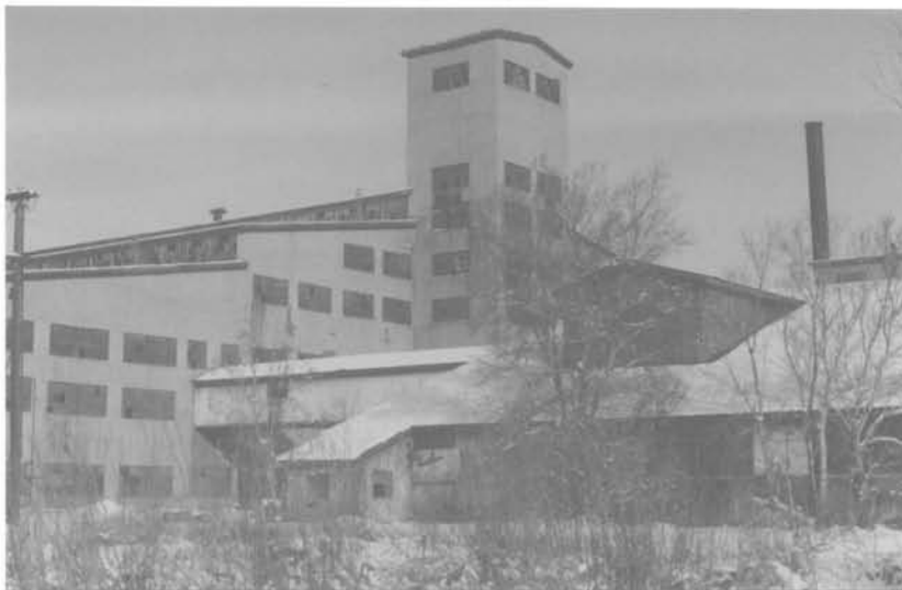
10. United States (U V Industries or Sharon Steel) mill and tailings near Midvale, Salt Lake County, 1982. Railroad (center) brought non-porphyry ores from Bingham district for processing by selective flotation. The mill also treated custom ores from other districts.
