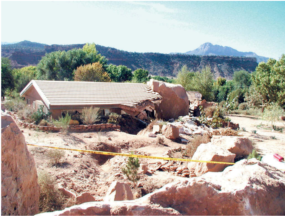
Figure 67. Block of Shinarump Conglomerate Member of the Chinle Formation that broke free from the cliff above Rockville, destroying a house and nearly crushing its occupant. Note gouge mark left by boulder as it rolled across the yard. Rockville is known for its homes nestled among large rock-fall boulders; here we have dramatic evidence that the process of cliff retreat continues today. Photo by Bill Lund, Utah Geological Survey.
