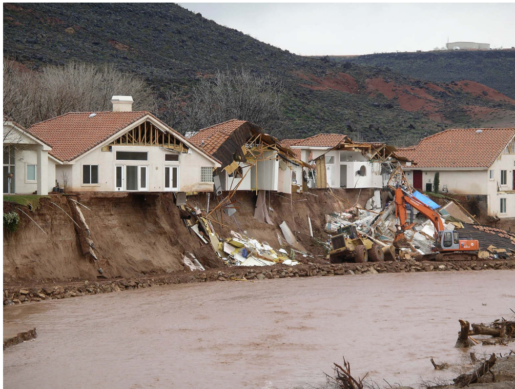
Figure 68. View northeast across the Santa Clara River to a subdivision off Indian Hills Drive, January 2005. Here, the Santa Clara River eroded laterally into terrace deposits, undermining and destroying several homes. While uncommon, large floods are a natural part of southwest Utah's geologic landscape, and building on floodplains and low terraces is not without risk.
