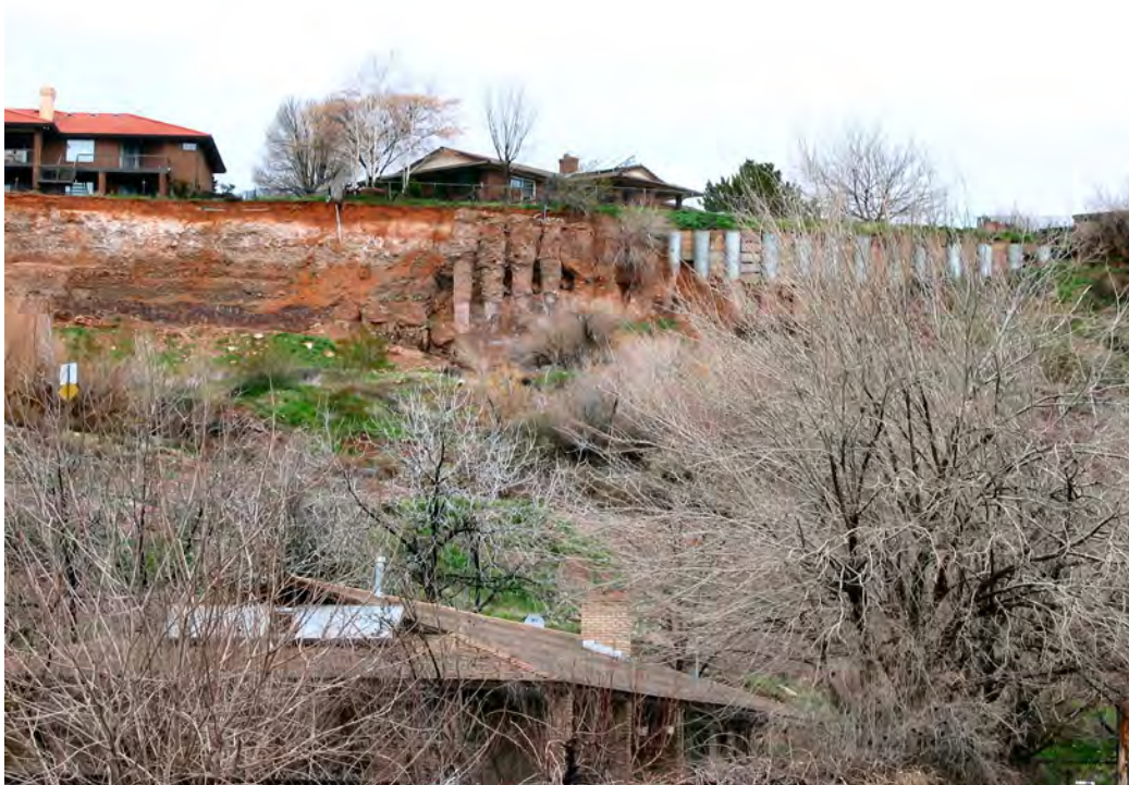
Figure 22. First recognized in the early 1980s, the Truman Drive landslide developed in the Petrified Forest Member of the Chinle Formation, and has remained intermittently active to the present; major periods of reactivation occurred in 1992 and again in 2002–03 (Lund and others, 2007b). In an effort to stabilize the main landslide scarp and prevent further damage to homes and utilities, large-diameter boreholes were drilled along the top of the slide, culverts reinforced with rebar were inserted in the boreholes, and the culverts were filled with concrete to create “soldier piles.” However, the landslide has continued to enlarge, destroying several of the piles. Large landslides in Petrified Forest strata are common, especially where exposed in steep hillsides protected from erosion by resistant cap rock or terrace gravels. The brightly colored swelling claystone of the member also exhibits a high shrink-swell potential (it expands when wet and shrinks upon drying), commonly leading to road and foundation problems.
