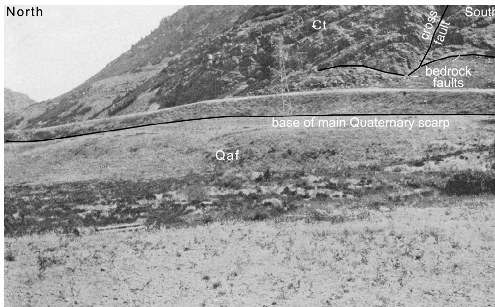
Figure 12. View looking east toward scarp along Wasatch fault zone (modified from Gilbert, 1928). Locations of abandoned bedrock fault traces, east-striking cross fault, and main active scarp indicated. Units are Ct - Tintic Quartzite, and Qaf - alluvial-fan deposits.
