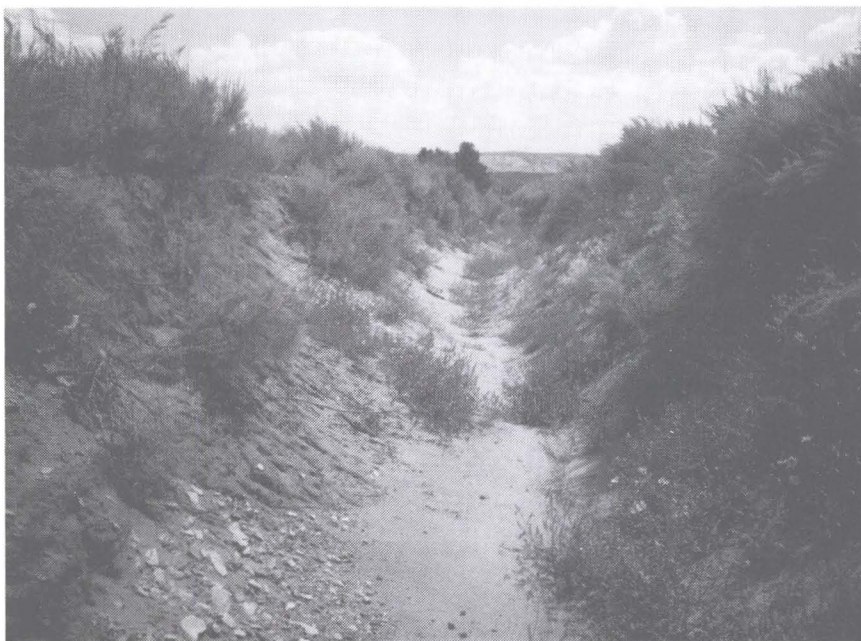
Figure 6. Very straight gullies in eolian sand were once roads. These roads were poorly located and collected water during floods. Proper siting of roads, with drainage "humps," can prevent this type of road damage.
