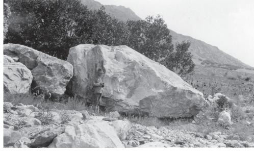
Photo taken September 1, 1925, of debris left by August 13, 1923, Willard flood, note man for scale. Largest boulder measures about 8 x 12 x 20 feet [~2.5 x 3.6 x 6 m]. Photo credit U.S. Geological Survey, photo by William Clinton Alden.
