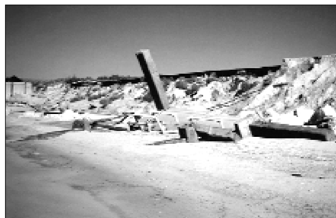
Figure 4. Debris from picnic facilities at north end of Antelope Island destroyed during mid-1980s rise of Great Salt Lake.
