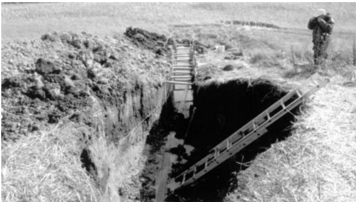
Figure 32. Photograph of the northern trench at Bloomington on the West Bear Lake fault zone. The widened part of the trench at the ladder is a section that caved in, when ground-water outflow from loose sands undermined the upper wall composed of cohesive silt and clay. This trench filled with water every 6 hours and had to be pumped out periodically in order to log the walls.
