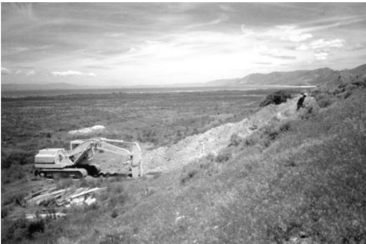
Figure 15. Photograph of the backhoe excavating the trench on the western fault scarp at North Eden Creek. View is to the north, with Bear Lake visible in the middle distance, and Merkely Mountain in the right distance.
