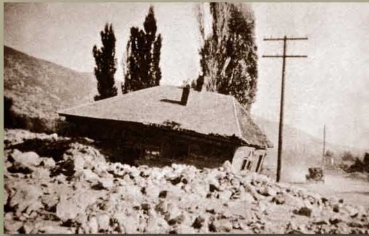
House moved by 1930 debris flow from Davis Creek near Farmington, Utah.
