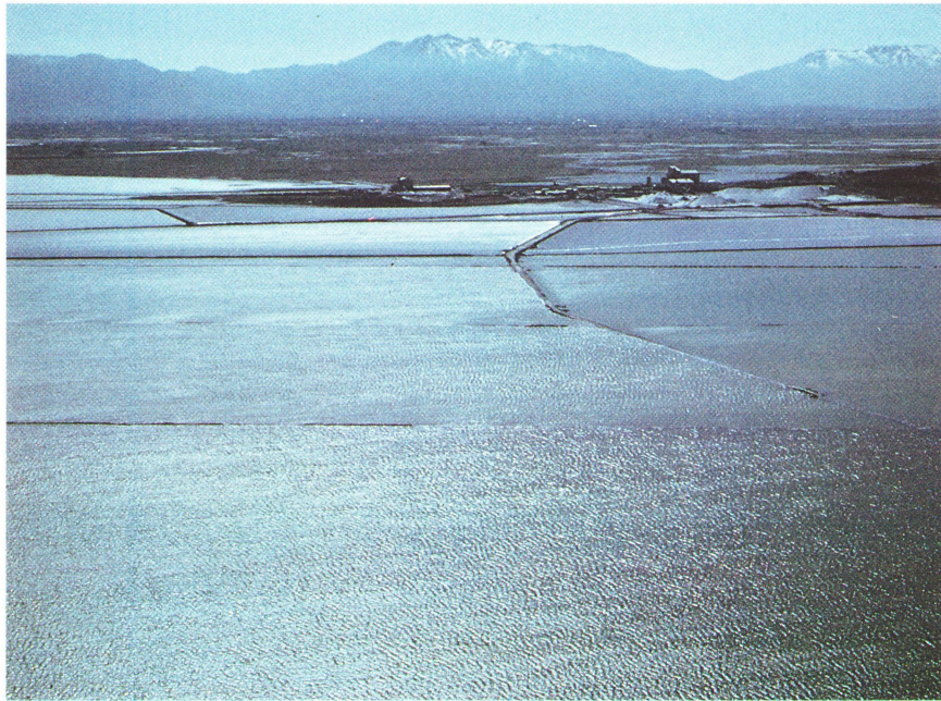
Flooded evaporation ponds. All of the salt industries on the Great Salt Lake are affected by fluctuating lake levels. Low lake levels require constructing canals and pumping brines to the ponds. High lake levels result in brine dilution and pond flooding. From 1983 to 1987, the lake level rose dramatically and industries looked for sources of more concentrated brine and new ponding areas which would be safe from the rising lake. Potential brine sources in Box Elder County that may be utilized include the more concentrated brine found at greater depths in the lake; the salt flat brines (muds and sediments of the Great Salt Lake Desert and mudflats surrounding parts of the Great Salt Lake that are saturated with saline water); and feasible solar ponding sites (large, flat areas with tight soil) that exist all around the north-western part of the lake.
