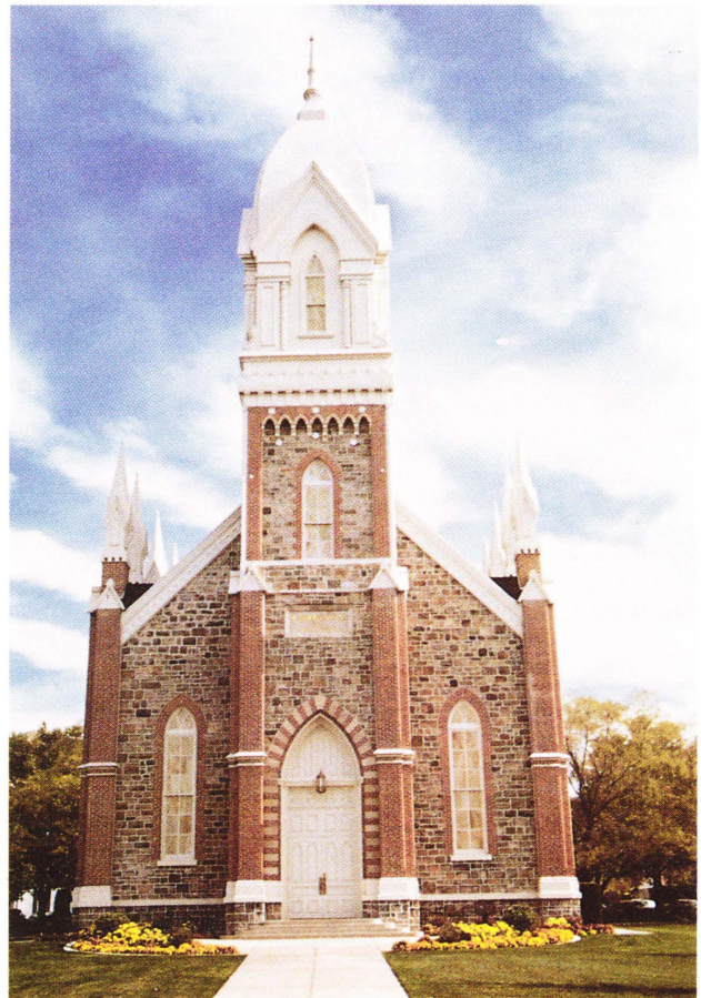
Local quartzite and sandstone, as well as brick, were used in the construction of this historic tabernacle in Brigham City. The pioneers often used a combination of brick and stone to construct buildings.
