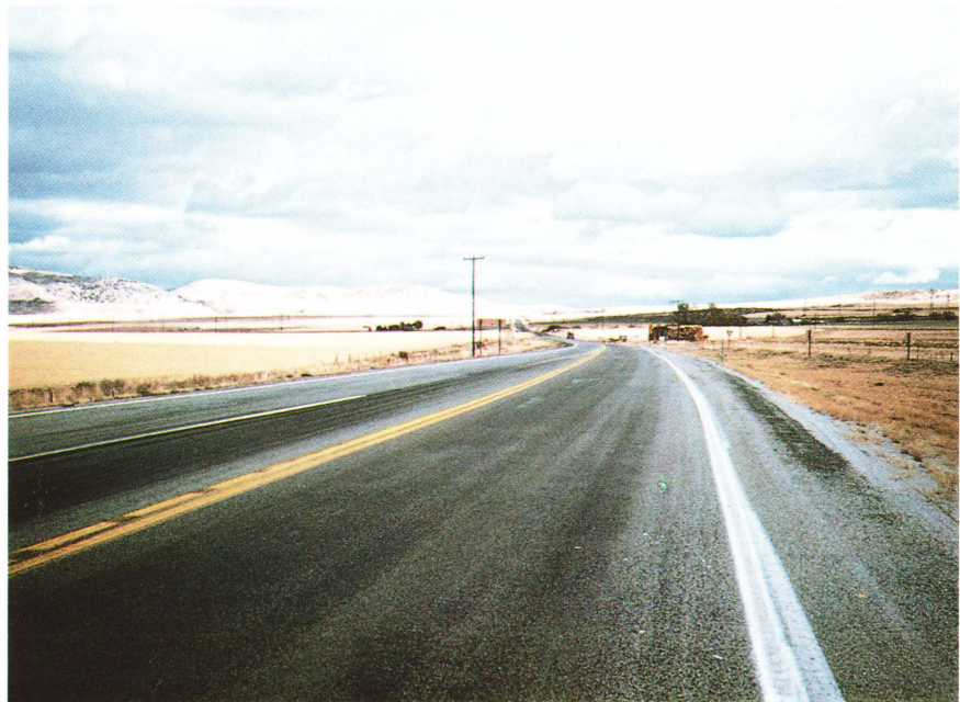
Road construction industry is a major user of crushed stone, sand, and gravel.
