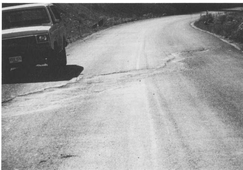
Figure 15. Payson Canyon landslide. From both road deformation and misalignment of center stripe, creep is evident on this 10-year-old landslide (slump) toe. This historic slide moved no more than this in 1983.
