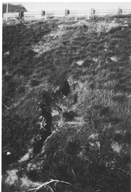
Figure 13. Salt Lake County, hydrogeologic effects; Upper: Collapse feature; Lower: Piping in interstate embankment.
