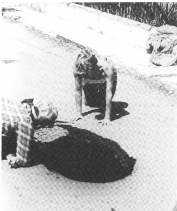
Figure 13. Salt Lake County, hydrogeologic effects; Upper: Collapse feature; Lower: Piping in interstate embankment.
