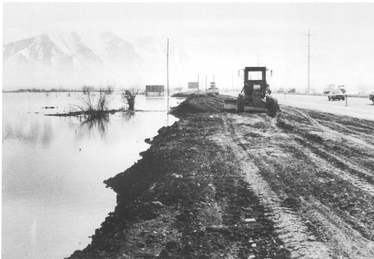
Figure 16. Embankment construction to protect I-15 from rising waters of Utah Lake (photo by Division of Comprehensive Emergency Management).
