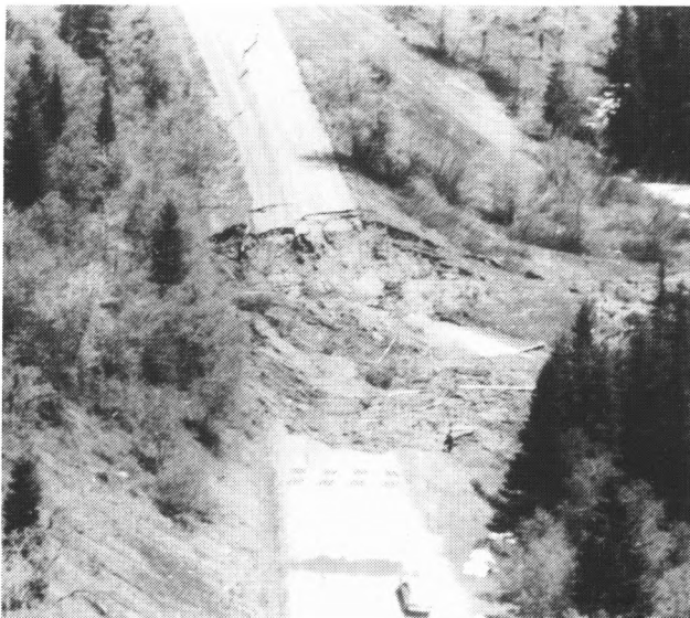
Figure 9. Slump taking out Hwy. 65 in East Canyon. Slide occurs in transition zone from cut to fill section of road. Note heavy tree growth, requiring relatively abundant water, directly upslope. Also note fracture with some vertical displacement indicating potential for considerable enlargement.
