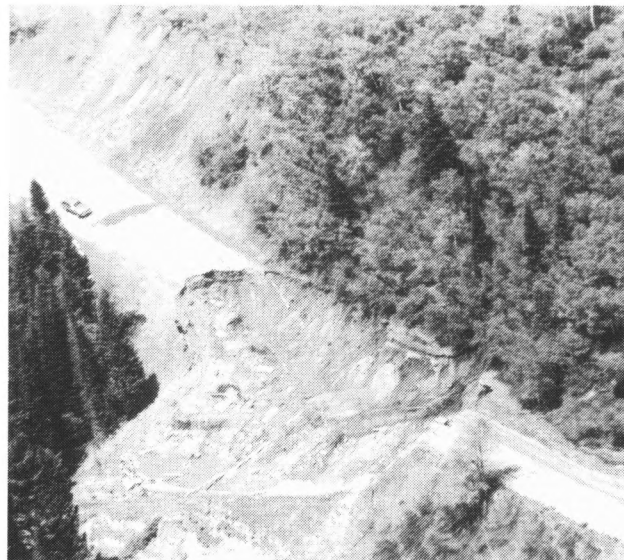
Figure 9. Slump taking out Hwy. 65 in East Canyon. Slide occurs in transition zone from cut to fill section of road. Note heavy tree growth, requiring relatively abundant water, directly upslope. Also note fracture with some vertical displacement indicating potential for considerable enlargement.
