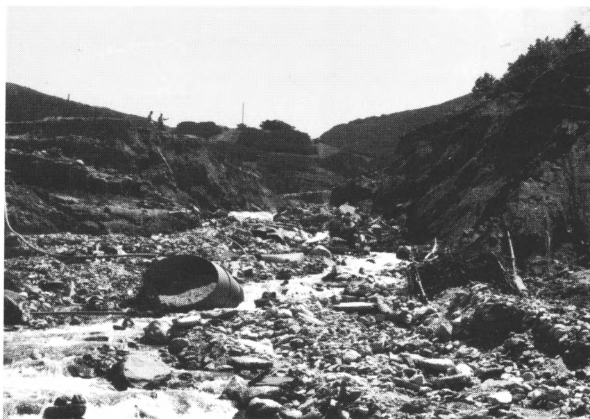
Figure 3. Drainage channels carrying debris flood loading in 1983 through cities of Bountiful and West Bountiful. Upper: Map of area. Lower: Stone Creek; collapse of embankment from debris floods (photo by Dan short).
