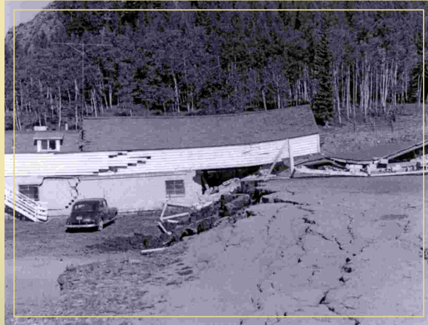
Fault scarp of the 1959 M7.6 Hebgen Lake, Montana, earthquake causing damage to barn (photo by I.J. Witkind).
