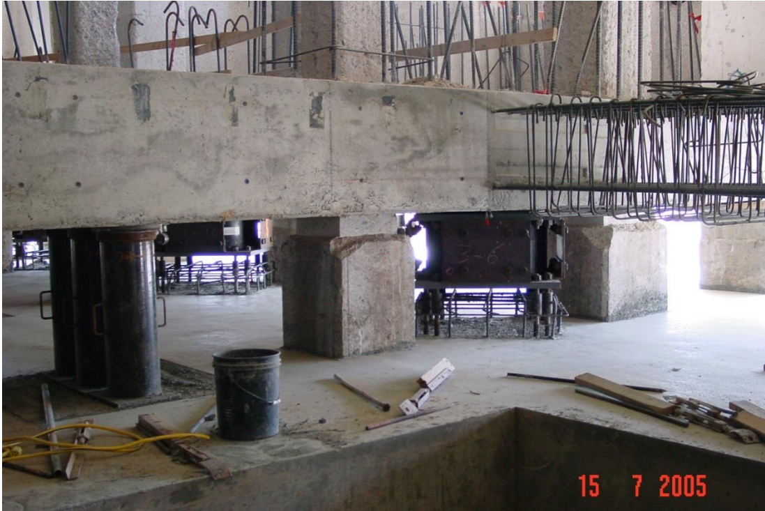
Figure 17. The Capitol building required temporary support to allow removal of the existing foundation and installation of the base isolation system. Photo courtesy Bob Carey.
