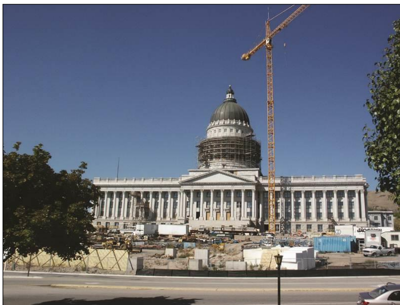
Figure 16. Construction to seismically retrofit the Utah State Capitol. Photograph taken September 2006 (UGS file photo).
