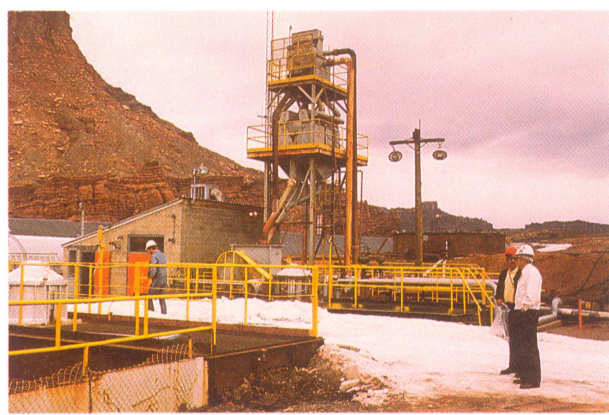
Potash plant at Cane Creek, near Moab (photo: H.H. Doelling).
