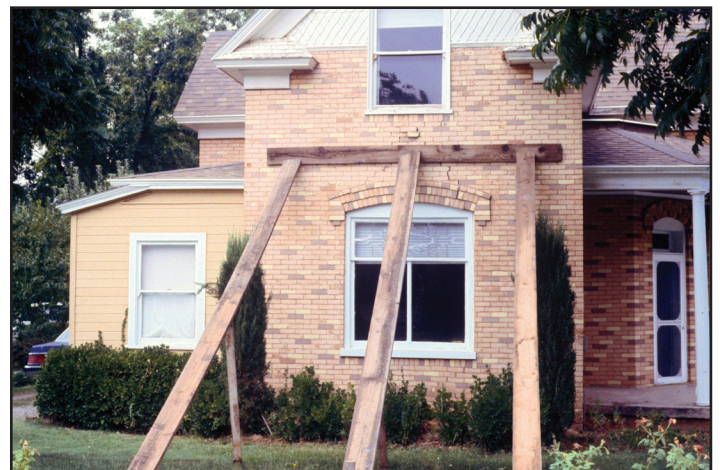
Bracing of an unreinforced masonry home damaged by the 1992 St. George earthquake. Cracks can be seen between the first and second story windows. Photo courtesy of the Utah Geological Survey.
