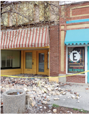
Damage in downtown Magna caused by the M 5.7 Magna earthquake of 2020. Photo courtesy of the Utah Geological Survey.
