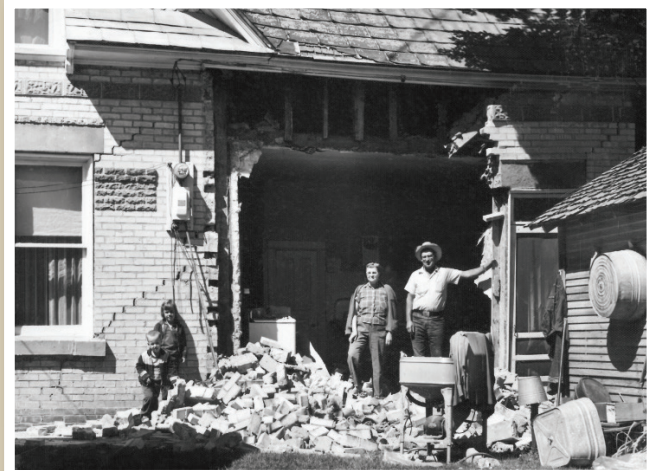
Damage caused by the M 5.5 Elsinore, Utah, earthquake of 1921 (above) and by the M 5.8 Richmond (Cache Valley) earthquake of 1962 (right). (Photos courtesy of, respectively, the F. J. Pack Collection, Special Collections Department, University of Utah Libraries, and Ariel D. Benson, Richmond, Utah)
