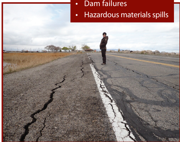
Cracks and road damage along the Great Salt Lake Marina access road likely from the 2020 M 5.7 Magna, Utah earthquake. Photo courtesy of the Utah Geological Survey.
