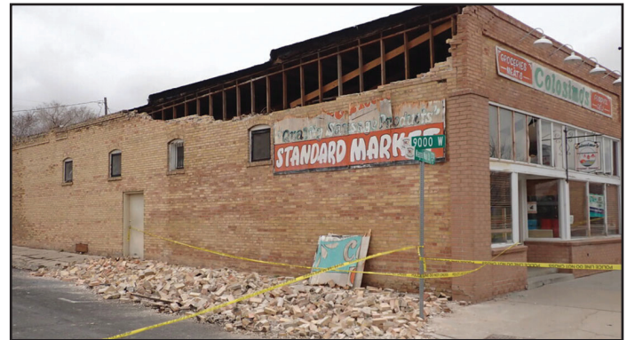
Structural damage to an unreinforced masonry building in downtown Magna caused by strong ground shaking from the Magma earthquake. Photo courtesy of the Utah Geological Survey.
