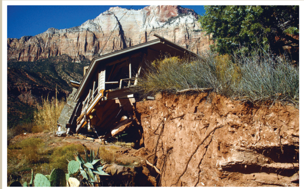
Home destroyed by the Springdale landslide, triggered by the September 2, 1992, M 5.5 St. George earthquake. Photo courtesy of the Utah Geological Survey.
