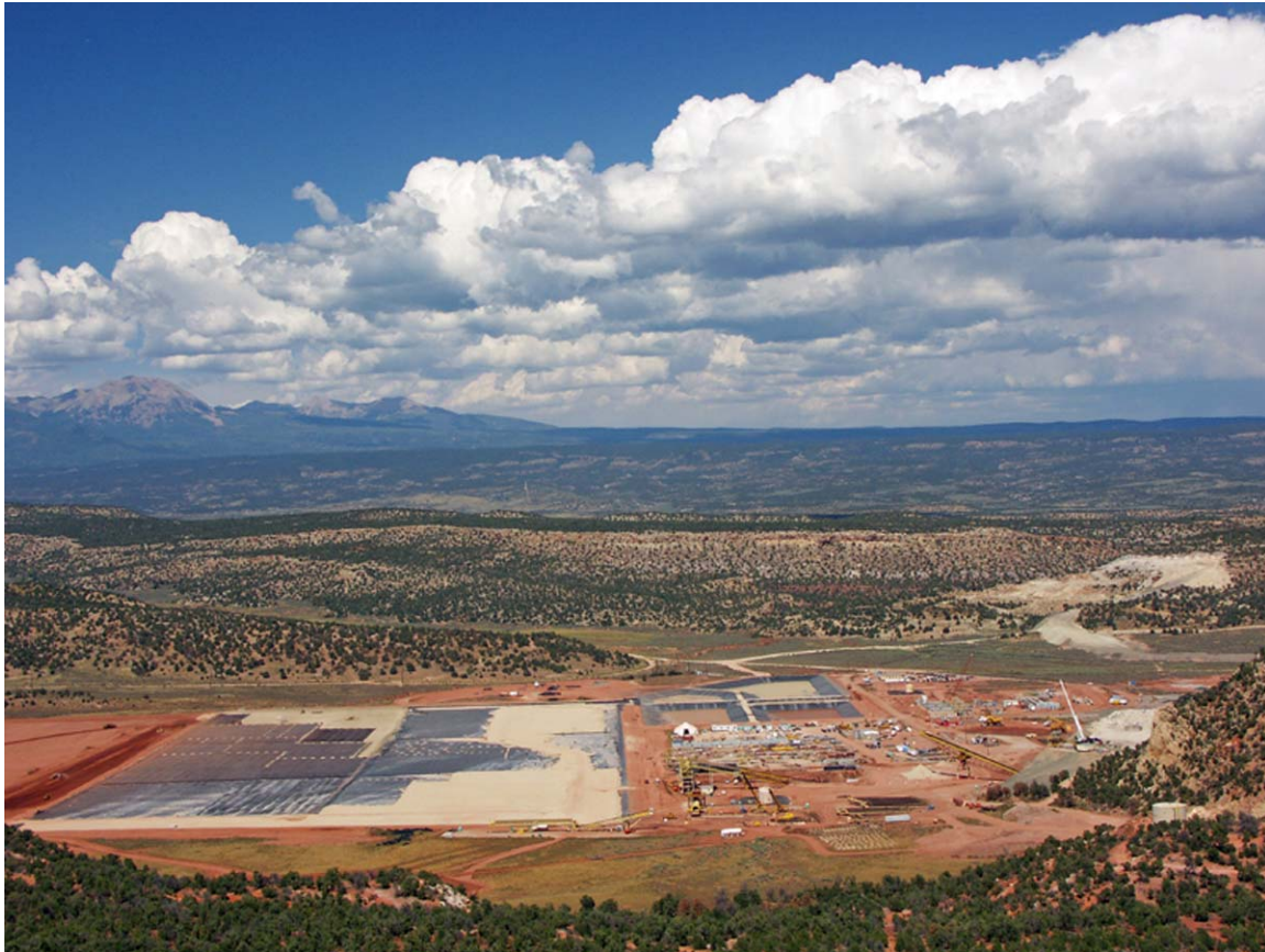
Figure 7. Constellation Copper Company's new Lisbon Valley copper mine and SX-EW plant, San Juan County, Utah.
