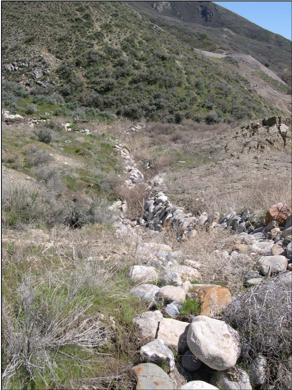
Figure 6. View of relatively intact, translated blocks near the middle of the landslide. Cobble-lined drainage ditch that was originally atop cut slope is translated downslope but relatively undeformed.
