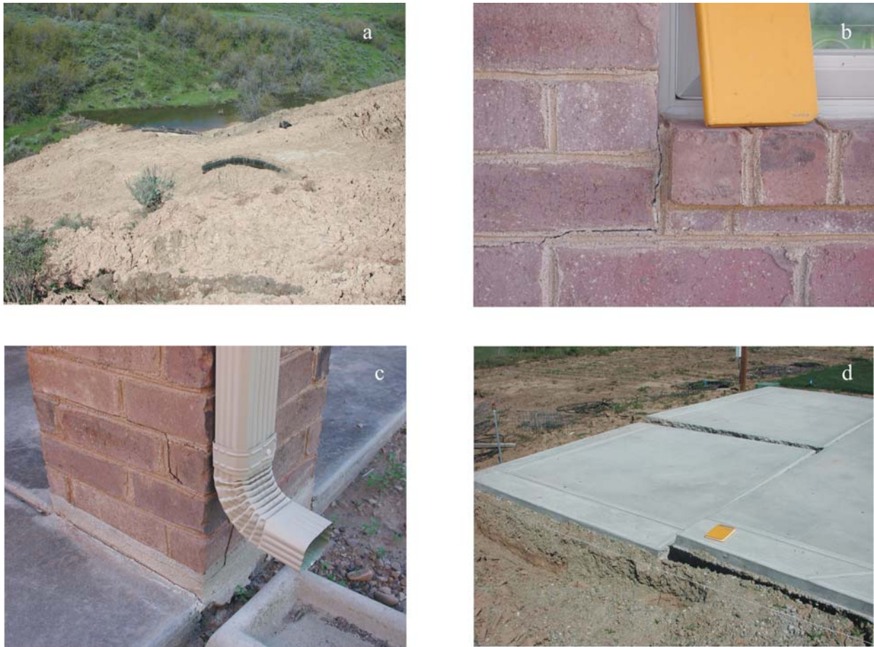
Figure 6. Damage caused by the Frontier Drive landslide. (a) Severed and segmented storm drain pipe downslope of lot 49. (b) Stair-stepping crack in wall of house on lot 49 ( 6815 N.). (c) Cracking of brick veneer of porch column of house on lot 49 caused by downslope movement (d) Damage to concrete patio or pad on lot 46 (6855 N.).
