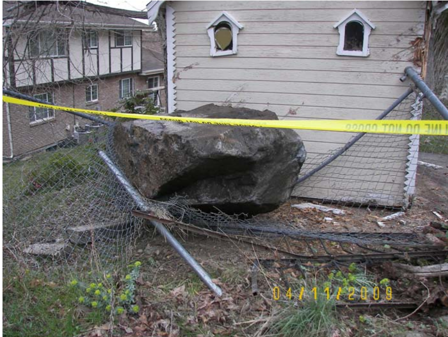
Figure 4. Rock-fall damage to chain link fence and playhouse at 1522 North 1550 East (Provo Fire Department photo). The rock size is estimated to be 2 x 4 x 3 feet.
