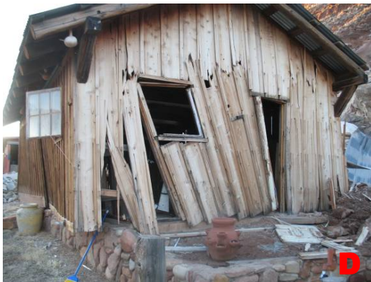
Figure 3. Impact area and damage to outbuildings. A. Large boulder (red arrow) at base of slope that broke up the rock fall. Yellow arrows show location of destroyed sheds. B, C. Destroyed sheds adjacent to impact area. D. Damaged workshop knocked off its foundation. E. Largest (9 x 6 x 5 feet) post-impact boulder that damaged a workshop (right) and shed (left).
