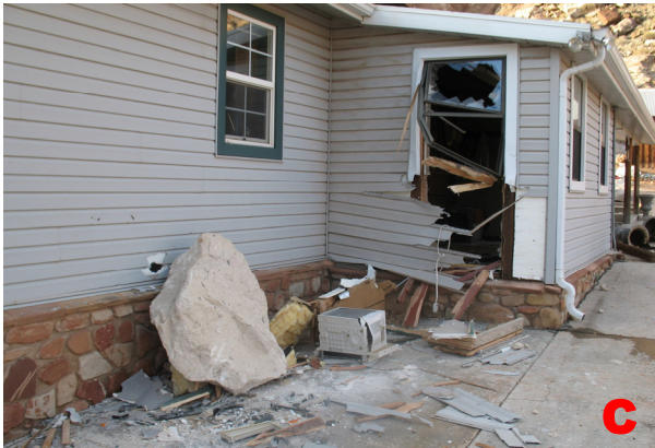
Figure 4. Rock-fall damage to the house at 274 Main Street. A. View downslope along path of rock that damaged the house. Narrowly missing a barbeque grill, the rock rolled through the entryway and mudroom on the left (east) side of the house. B. Looking through the mudroom where the boulder broke through a glass door, which is still on its hinges, and exited through an exterior wall and window. C. After exiting the mudroom, the rock collided with a parked car and came to a rest. The rock, estimated to be 3.5 x 3 x 1.7 feet, was later moved up against the house when the damaged car was removed.
