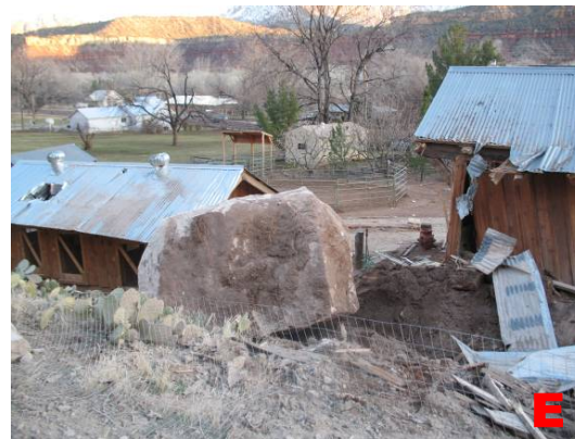
Figure 3. Impact area and damage to outbuildings. A. Large boulder (red arrow) at base of slope that broke up the rock fall. Yellow arrows show location of destroyed sheds. B, C. Destroyed sheds adjacent to impact area. D. Damaged workshop knocked off its foundation. E. Largest (9 x 6 x 5 feet) post-impact boulder that damaged a workshop (right) and shed (left).
